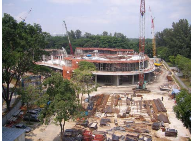
Level 3 floor slab taking shape
