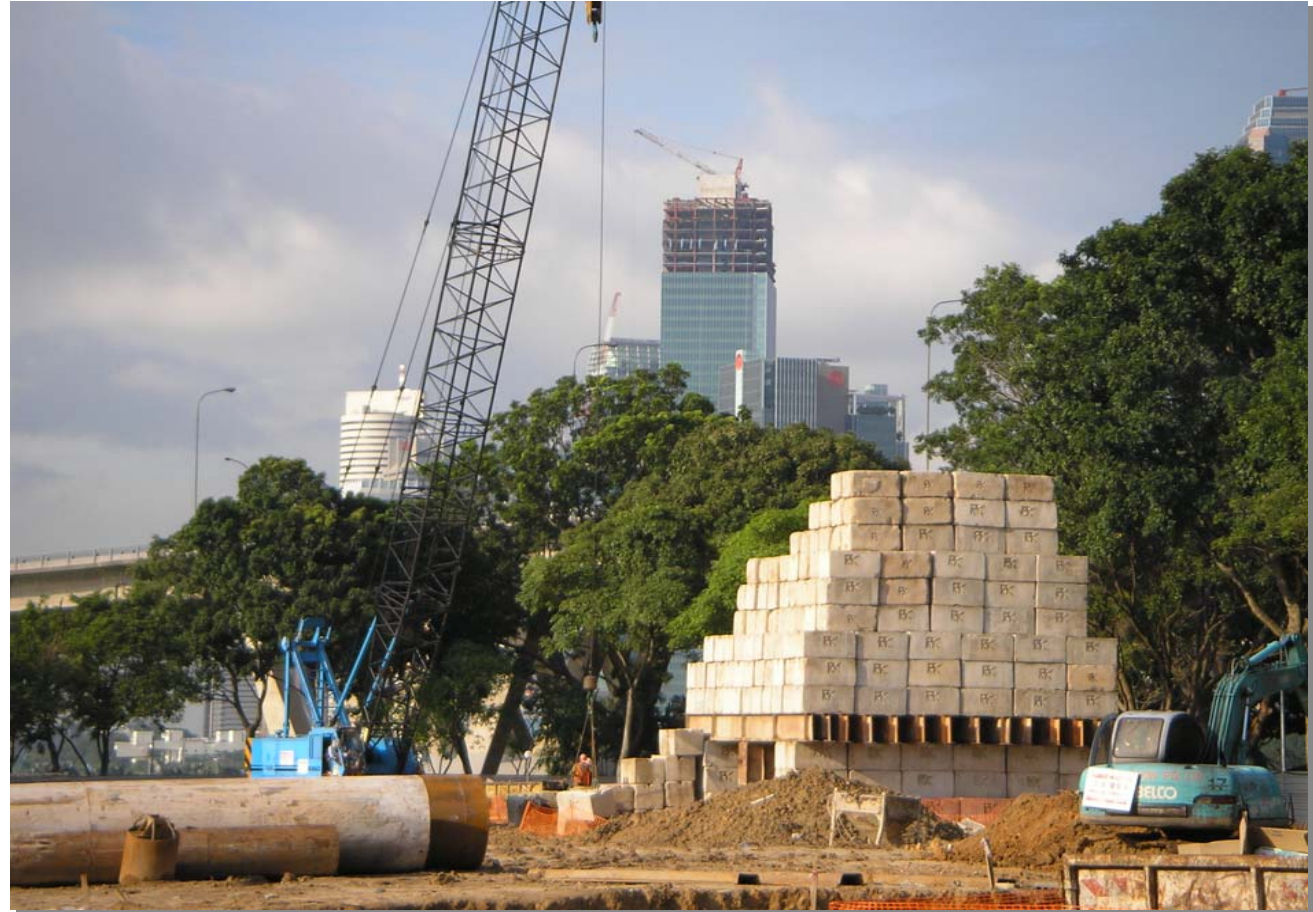
Piling Load Test
