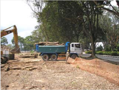
Land Clearing Begins
