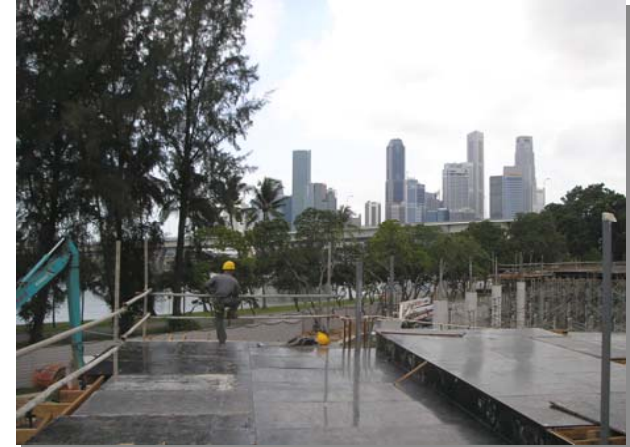
View from Level 2 formwork base for concrete
