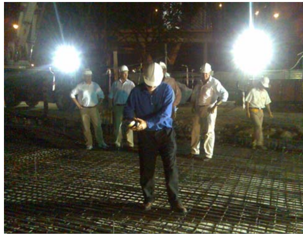
Sake pouring ceremony prior to final ground floor slab concrete pour
