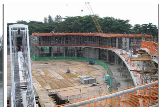
Central courtyard crane working area
