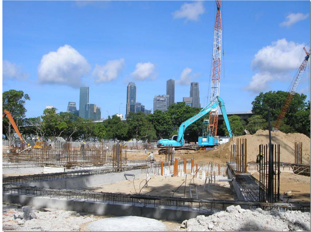
Work begins on Ground Floor slab
