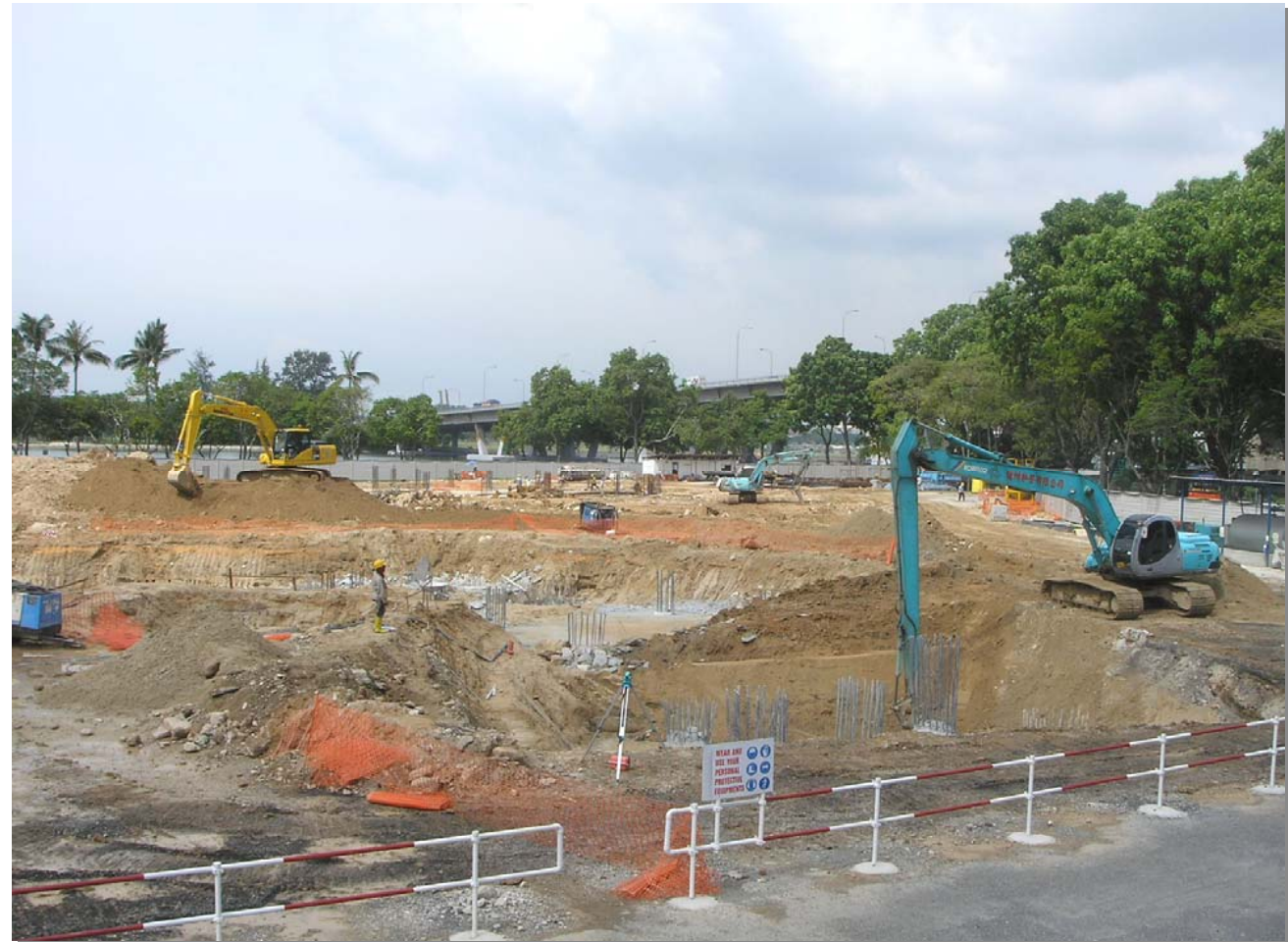
Work begins on the foundations for the Long Support Cable base
