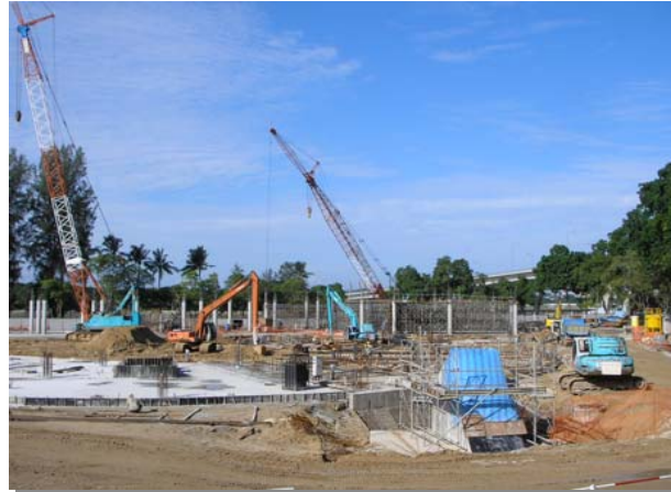
Ground floor slab nearing completion
