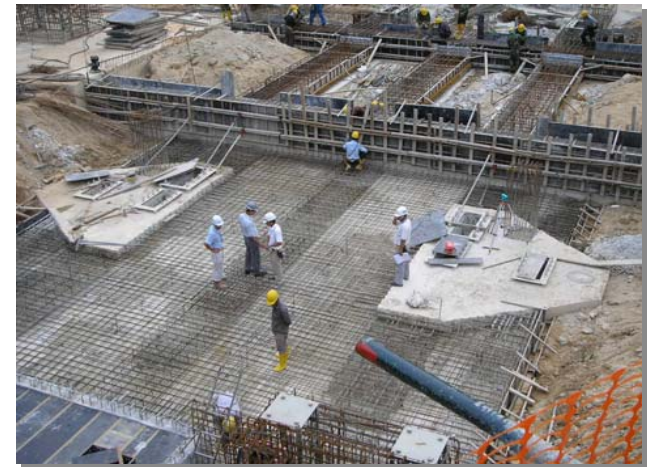
Concrete base plates for GOW legs
