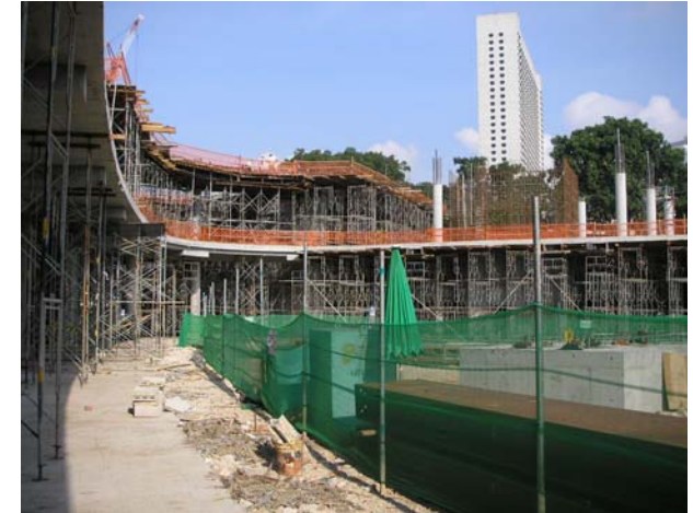
View from the central courtyard
