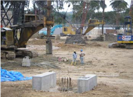
Preparing Pile Caps
