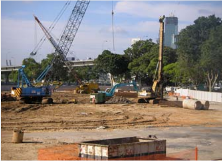
The First Test Pile
